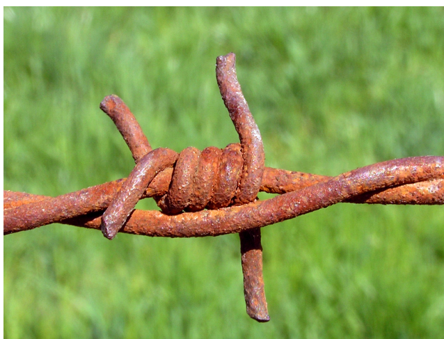
Figure 17.2 “Rusted Barbed Wire.” The rusting of barbed wire occurs over many years.
