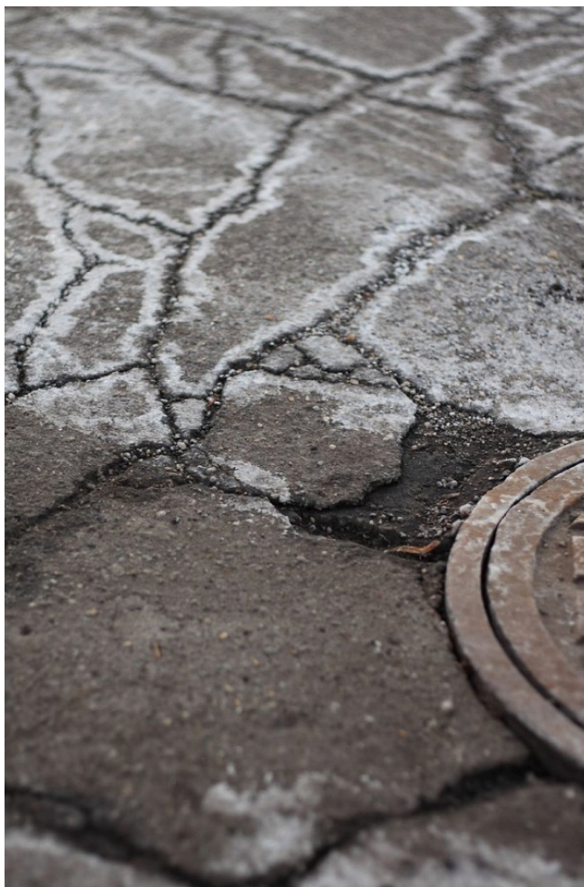
Figure 11.2 “Salt and Safety.” Salt or other compounds take advantage of the freezing point depression to minimize the formation of ice on sidewalks and roads, thus increasing safety.
